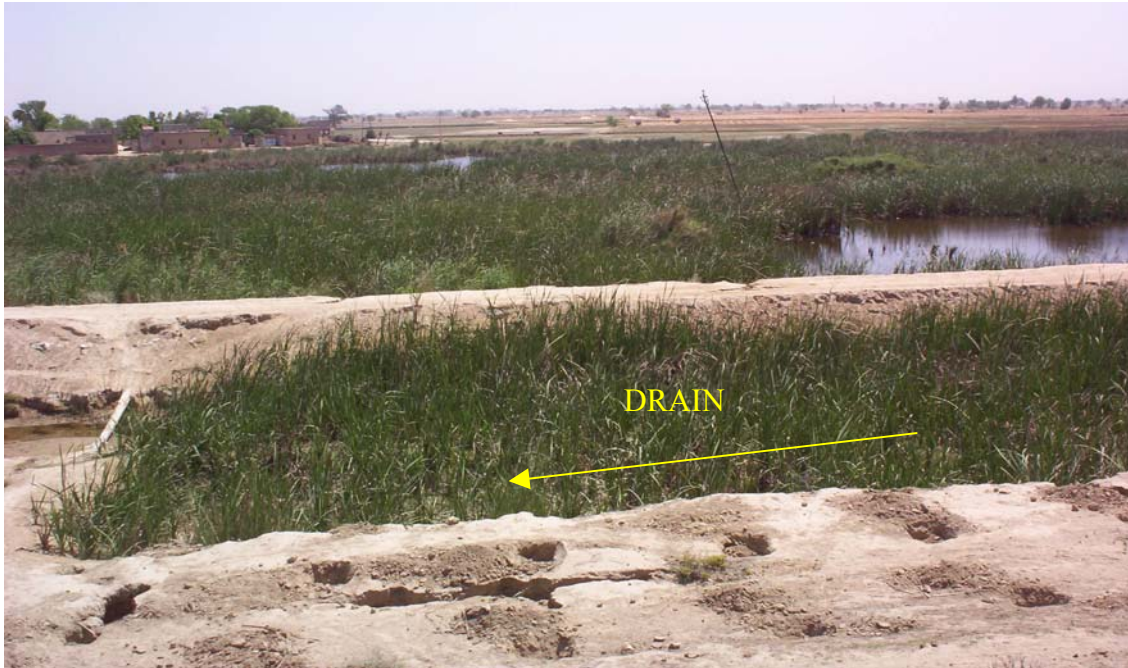
Figure 11. Drainage congestion due to wild grass growth. Village: Theri, Tehsil: Gidderbaha.
