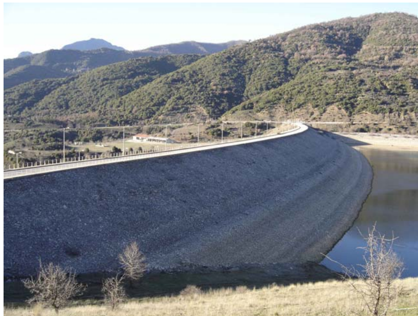
Figure 2: Upstream view of the Mornos dam and its surroundings.
