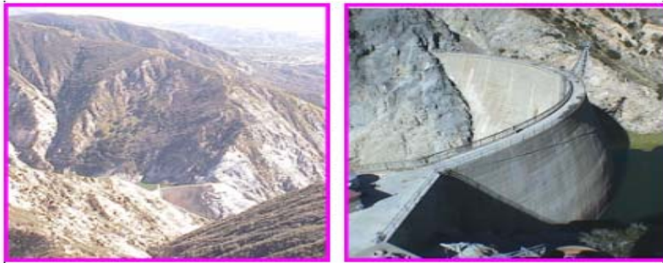
Figure 4 : Pacoima dam view
